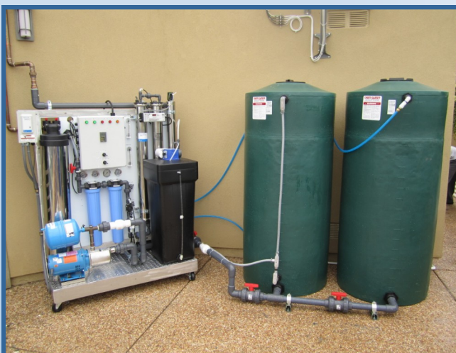
Actual whole house system installed in a home at Solana Beach, California. Included in this unit is a silent water cooled pump system, alkaline boost, Aquafer scale preventer and 30 gpm re-pressure pump.
